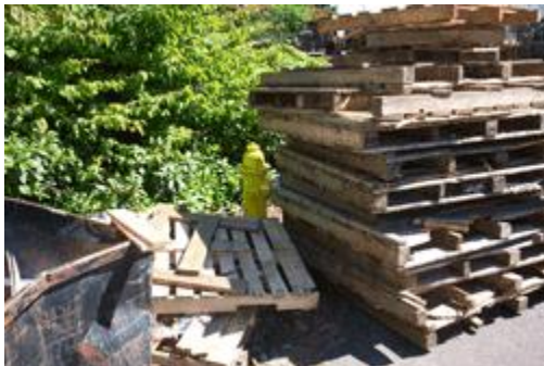
Fire hydrant is blocked by idle pallets.
